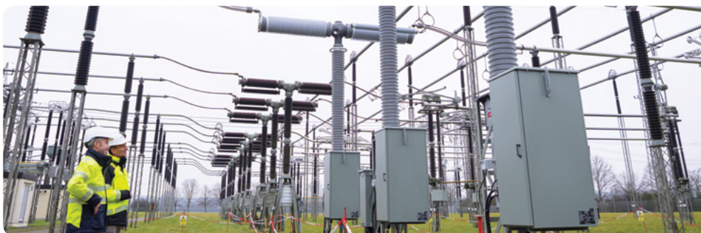
World's first SF 6 -free 420 kV live tank circuit breaker – TenneT Germany
