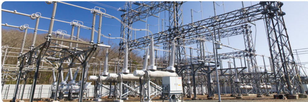
World's first SF 6 -free 420 kV dead tank circuit breaker – Eversource
