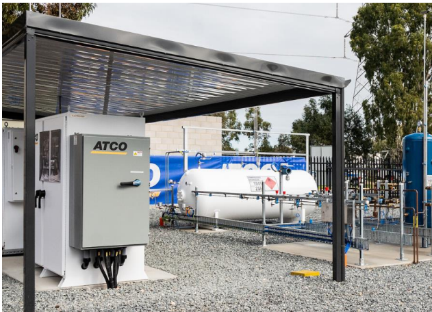
Fig. 2. 260 kVA controllable hydrogen electrolyser (front left) and 30-bar high-pressure hydrogen storage vessel (centre) [3].
