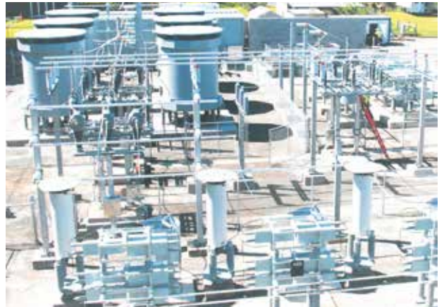
Directly connected SVC
